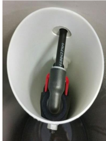
Brine well & fitting with overflow device
