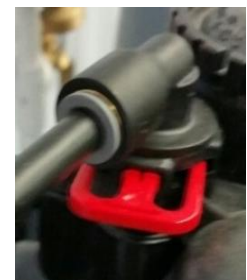
Brine line connection
