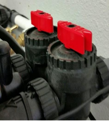
By-pass valve in closed position.
