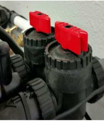
By-pass valve in closed position.
