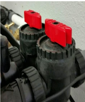
By-pass valve in closed position.
