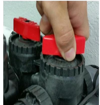
Slowly open valve inlet 1/3 to fill tank.
