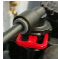
Brine line connection
