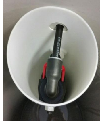
Brine well & fitting with overflow device
