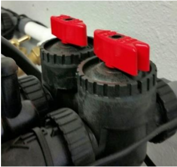
By-pass valve in closed position.
