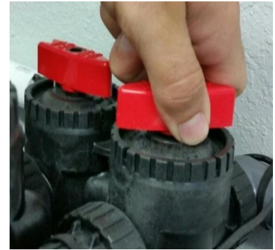
Slowly open valve inlet 1/3 to fill tank.
