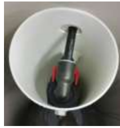
Brine well with overflow prevention device.
