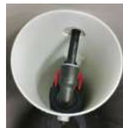
Brine well with overflow prevention device.
