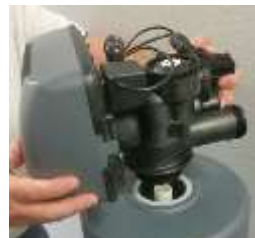
4. Install valve on mineral tank.
